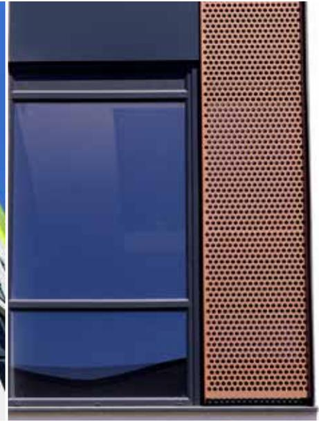
First off, the 2000 windows delivered an engaging lesson in physics. Their versatile design allows trickle ventilation when opened on the tilt. Or creates full purge when opened along the vertical frame axis.
