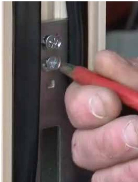
Once the door is operating correctly, fix the remaining screws to the hinges and rollers.
