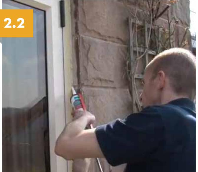
The door can now be fully sealed with silicone and cleaned.
