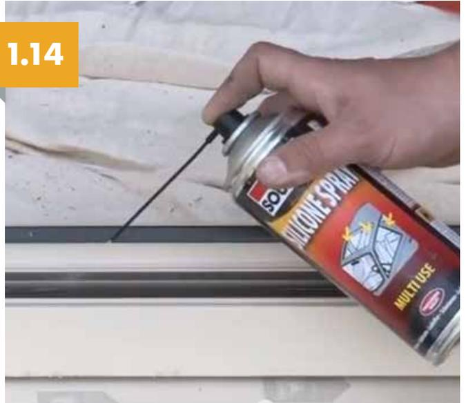
Ensure the top & bottom roller cases are free from debris or obstacles which may impair the function of the product. We recommend that silicone spray is used to speed up the 'bedding in' period of the rollers, ensuring a smooth effortless action, spray both the head & the cill aluminium channels.
