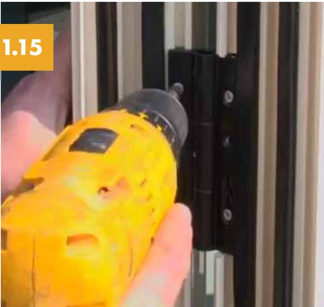
Hinge adjustment is achieved by loosening off the 2 screws on each leaf and then sliding the adjuster peg to suit, once the lateral adjustment has been made please ensure to carefully tighten the screws. (5mm lateral & 2mm height adjustment available per hinge).
