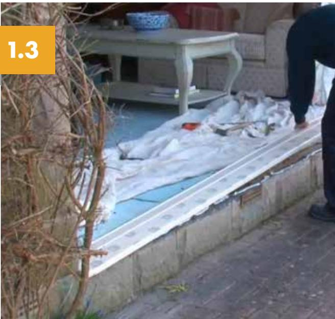
Apply a generous bead of silicone across the bottom of the aperture to sit the base cill on and fix the cill to the aperture ensuring that it is level.
