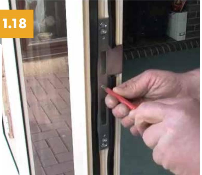
Traffic door keep adjustment is achieved by using the screws, which simply need to be loosened, in order to give inward and outward adjustment. Once the keep is in the correct position carefully retighten the screws.
