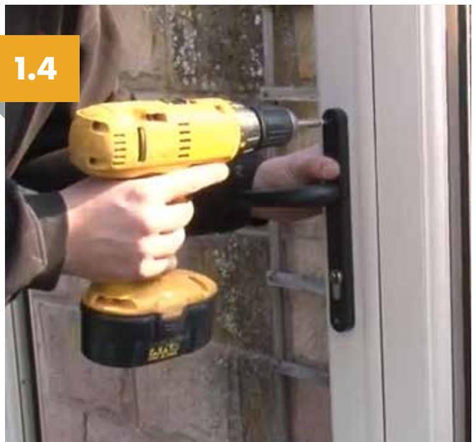
Fix the traffic door handle & lock cylinder to the door.
