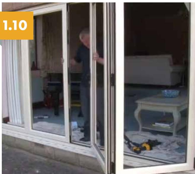
Check that the sashes operate correctly before the glazing begins.
