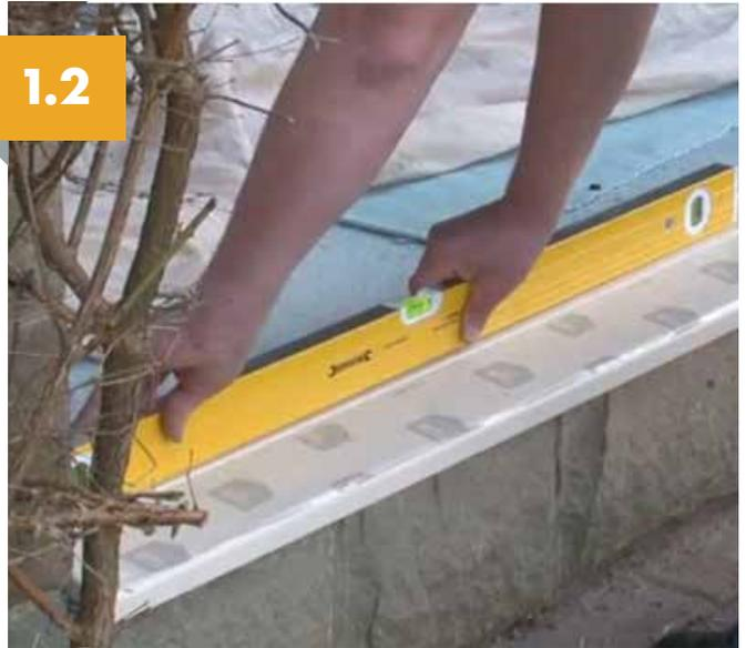
Offer the base cill into the opening, check the cill is level across its overall length (maximum deviation is 3mm).
