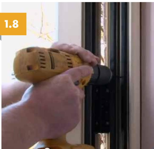
Fixings in the jambs should be fitted through the centre line of the euro groove. The suitable fixings for this installation are available from all Eurocell building plastics depots.
