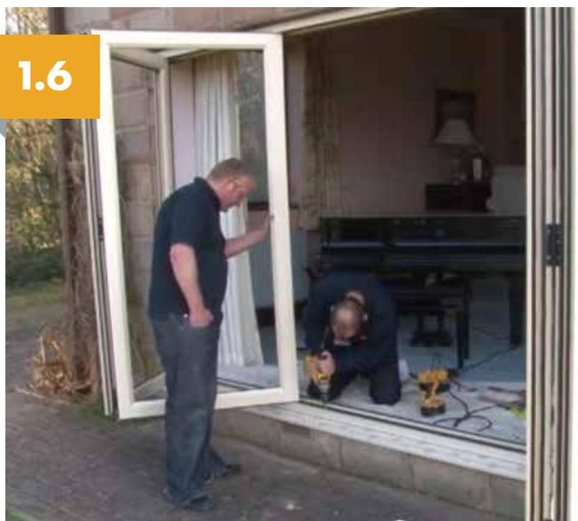
Once in the correct position and the door is plumb and square without twist, you can begin fixing the door into the opening, using appropriate fixings (not supplied). When fixing down to the cill, ensure that screws are sealed to prevent water ingress. Also seal across the cill below the door jambs to prevent water tracking across the cill.
