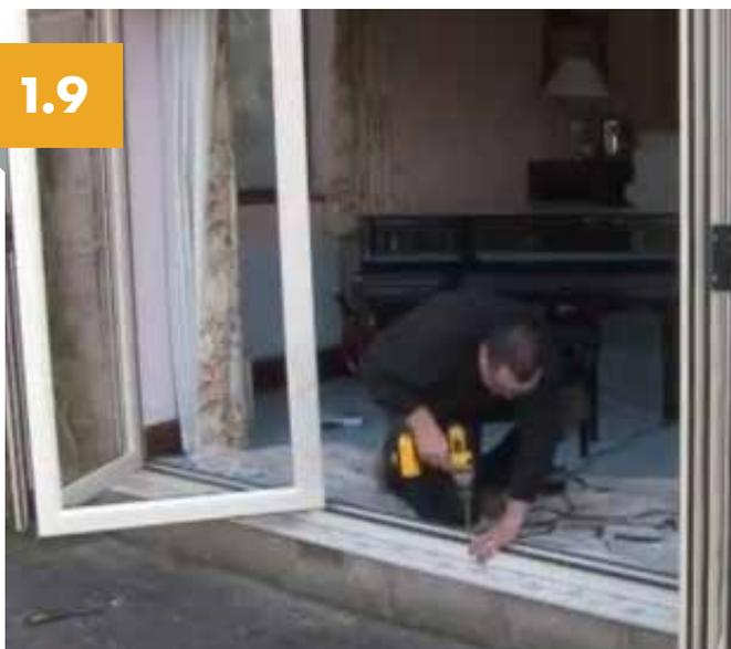
The fixings in the head and cill should sit as flush as possible to enable the rollers to easily pass over the fixings but it is important that these are not over tightened as this will distort the aluminium track and prevent the door from operating correctly.
