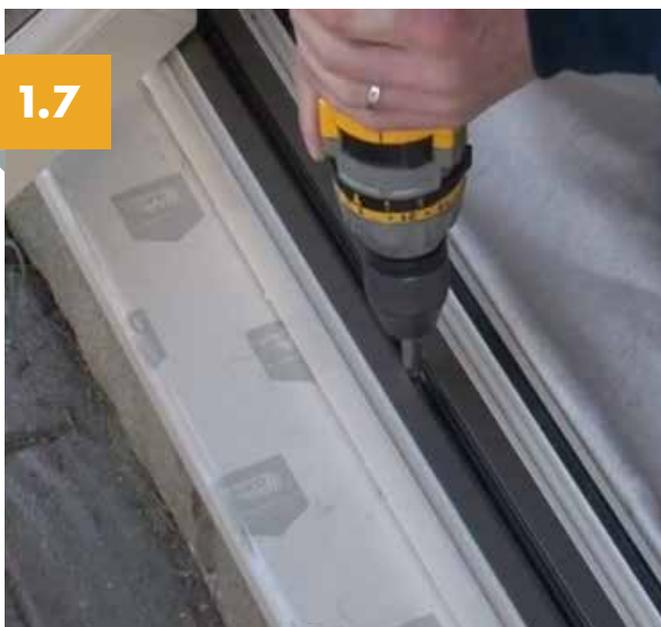
Fixing distances: corner fixings shall be a minimum of 150mm and a maximum of 250mm from the corner. Intermediate fixings shall be at centres no greater than 600mm.
