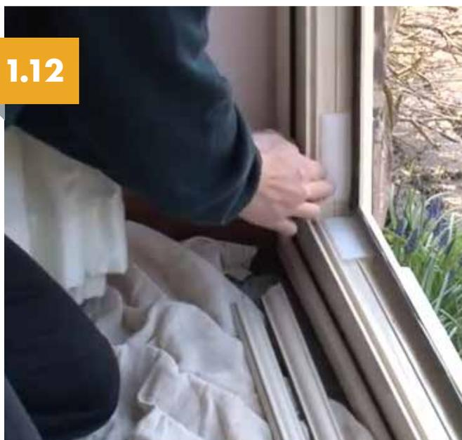
Fit the glass and pack appropriately. All sashes must be toed and heeled to ensure an equal and parallel sight line between the head of the sashes and the outerframe. When the glass is fully packed out, re-bead placing the beads in their original locations.
