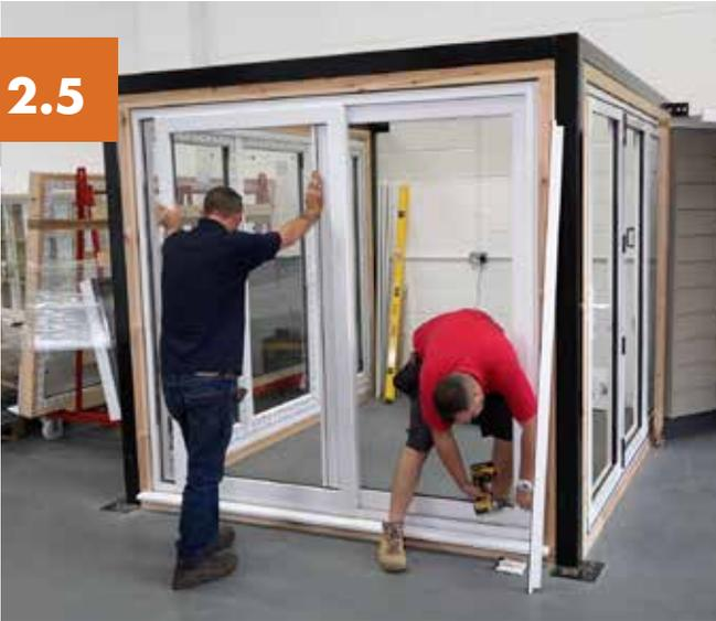
Remove old fixings and break the external silicone seal with a blade.
