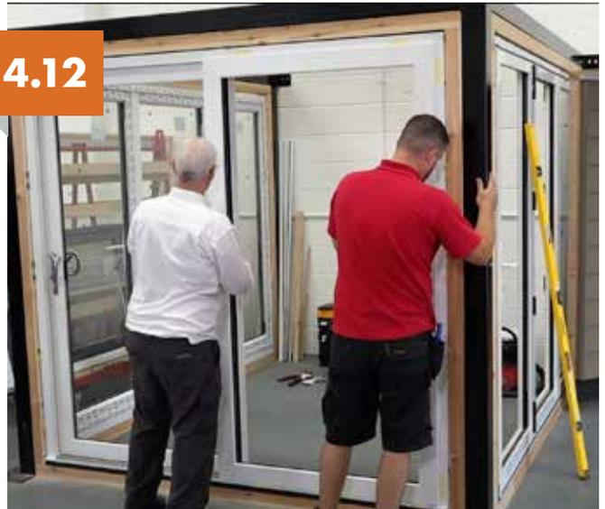
Slide sash back across and fix sash to frame.
