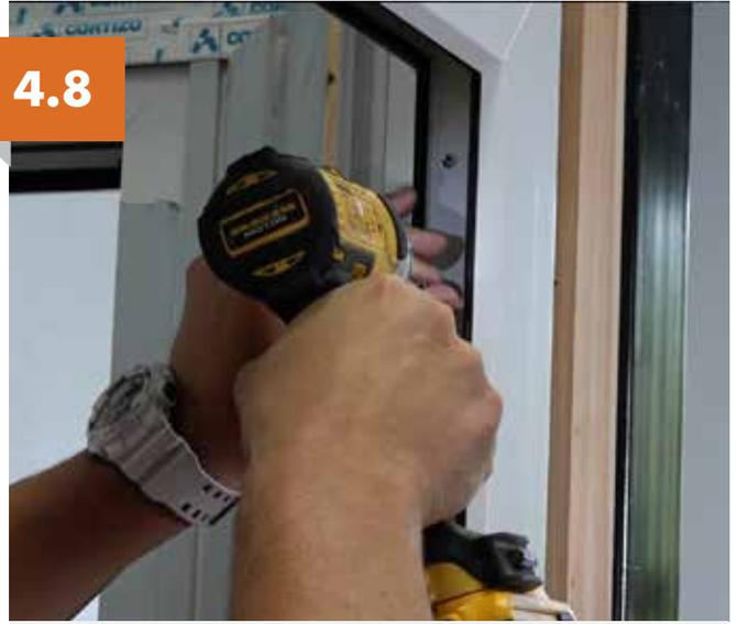
Remove screws from fixed sash and slide back away from frame.
