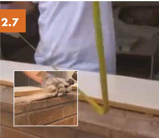
Check that mortar bed has sufficient clearance, if not remove it.
