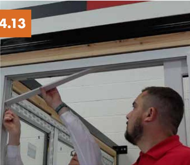
Peel trim down from slider head and fix other side.
