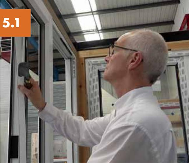
Remove the beads to allow for glazing. Mark each bead with location to make refitting easier.
