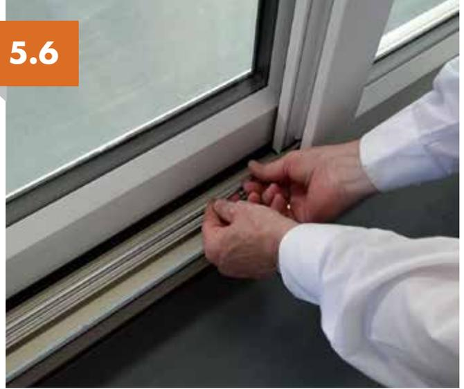
Adjustment – once the door is set, check to make sure the sash is square on the track. Use an allen key for adjustment of up and down movement if necessary.
