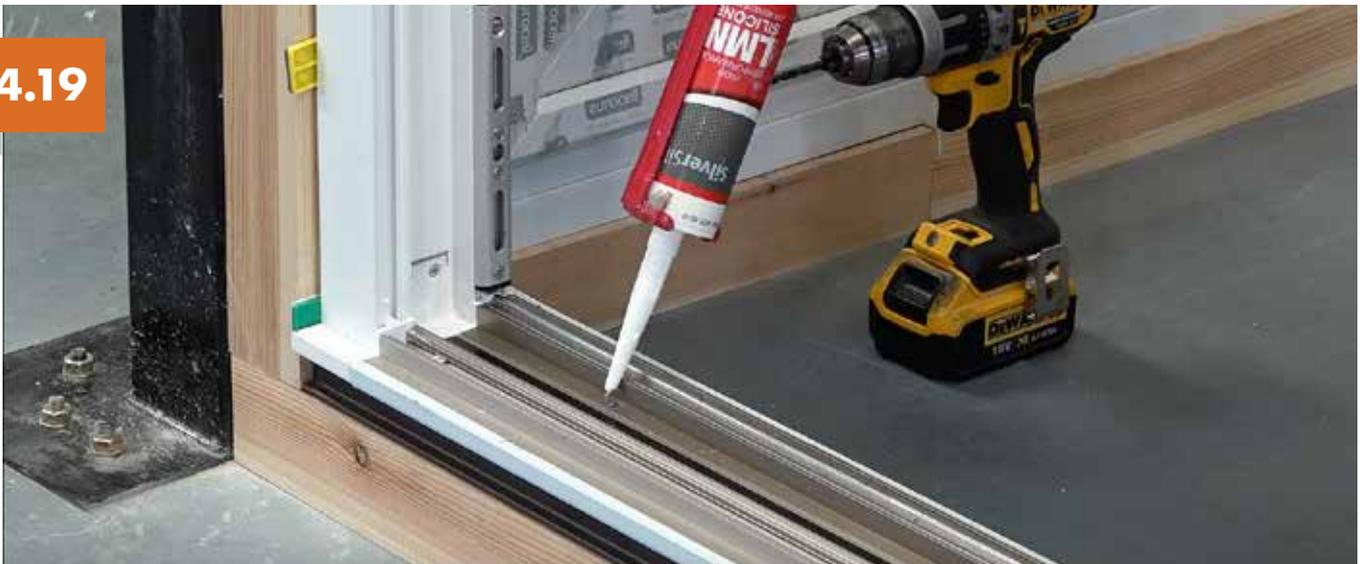
Mastic in the hole to seal the head of the screw.
