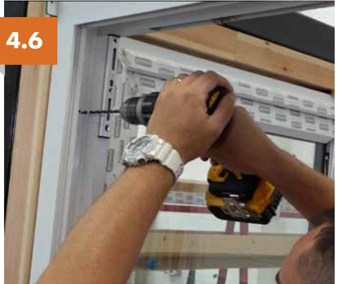
Drill clearance hole for relevant fixing.
