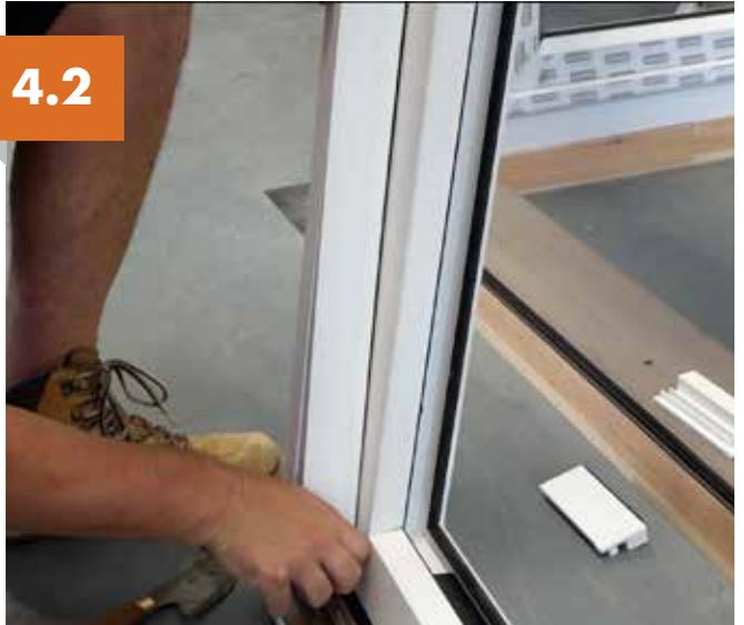
Remove all covers to allow for frame fixings; tops, bottom and sides.
