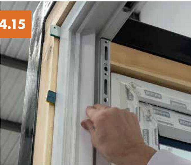
Slide in on an angle so the foot positions under the pip and clip the outside into position. You will hear a click when fitted correctly.
