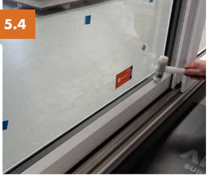
When putting the beads back in – tap from the sides to the middle to ensure the bead is tight into each corner, using a nylon head mallet.
