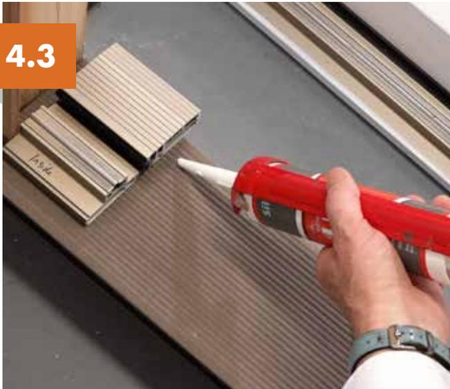
Put 2 lines of bed mastic to the base (front and back) to create a water tight seal to the base of the door.
