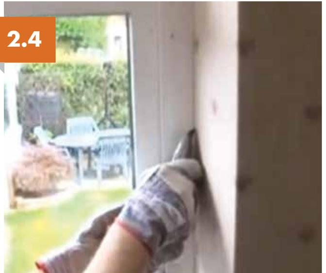
Run a sharp blade around the inside perimeter of the door to break the bond between frame and the plaster. This will also minimise the damage to any interior decoration.
