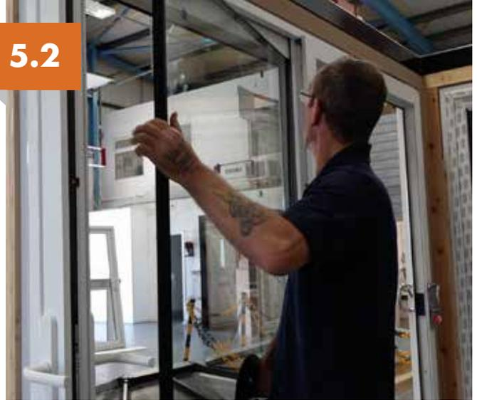
Lift the glass using a glass lifter, position lifter in centre of pane. Allow a slight angle on interlock side when offering up into position.
