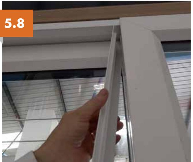
When 100% happy that the door is set, position the interlock covers in place. Tap the back in first down the length then tap down the front face.
