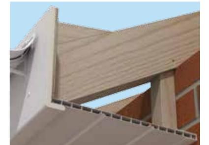
9mm capping board and 300mm hollow soffit board
