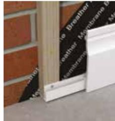
Always start the installation at the base, creating a level situation before fitting a starter trim.
