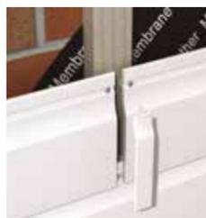
Butt joint trims can be used instead of joint trims providing they are staggered and fitted where a batten is located
