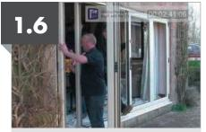
Once in the correct position and the door is plumb and square without twist, you can begin fixing the door into the opening, using appropriate fixings (not supplied). When fixing down to the cill, ensure that screws are sealed to prevent water ingress. Also seal across the cill below the door jambs to prevent water tracking across the cill.
