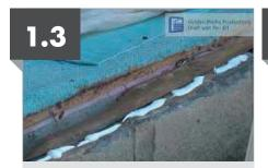
Apply a generous bead of silicone across the bottom of the aperture to sit the base cill on and fix the cill to the aperture ensuring that it is level.
