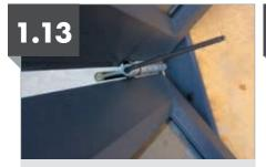
Roller hinge adjustments can be made. For further details refer to hinge adjustment details on the following page.
