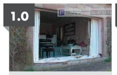
Before installing the Aspect door, the structural opening should be cleared of all dust and debris, and a check made to ensure the D.P.C is in position and is undamaged.
