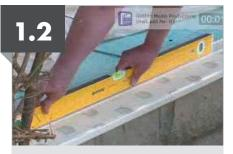
Offer the base cill into the opening, check the cill is level across its overall length (maximum deviation is 3mm).
