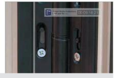
Hinge adjustment is achieved by loosening off the 2 screws on each leaf and then sliding the adjuster peg to suit, once the lateral adjustment has been made please ensure to carefully tighten the screws. (5mm lateral & 2mm height adjustment available per hinge).
