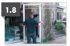
The fixings in the head and cill should sit as flush as possible to enable the rollers to easily pass over the fixings but it is important that these are not over tightened as this will distort the aluminium track and prevent the door from operating correctly.
