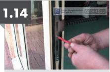
Traffic door keep adjustment is achieved by using the screws, which simply need to be loosened, in order to give inward and outward adjustment. Once the keep is in the correct position carefully retighten the screws.
