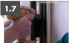
Fixing distances: corner fixings shall be a minimum of 150mm and a maximum of 250mm from the corner. Intermediate fixings shall be at centres no greater than 600mm.
