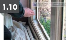
Fit the glass and pack appropriately. All sashes must be toed and heeled to ensure an equal and parallel sight line between the head of the sashes and the outerframe. When the glass is fully packed out, re-bead placing the beads in their original locations.
