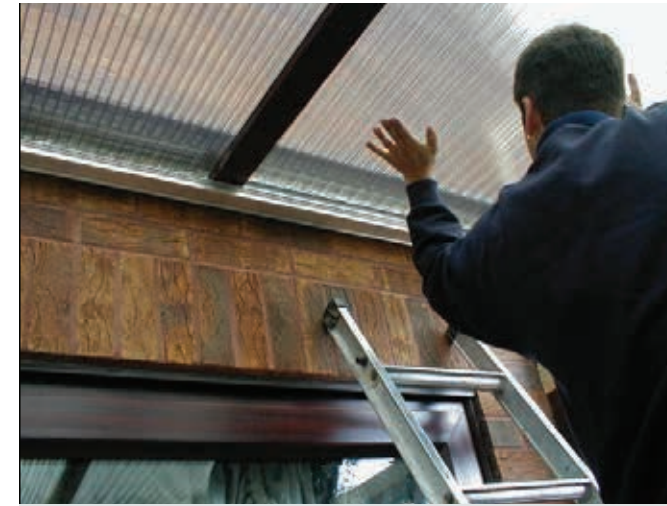
10) Slide the Glazing onto the Rafters and into the Ridge/Wall Plate Glazing Trims.
