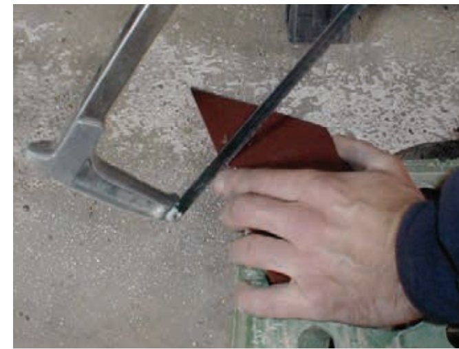
13) The Ring Beam End Cap can now be fitted. To fit the End Cap, first cut down the capping to suit the pitch of the roof as shown.
