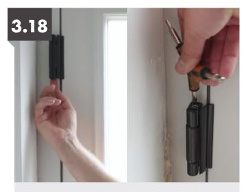
The hinges can also be adjusted up and down. Ensure the allen key underneath is fully loosened off, to adjust the hinge up or down, use the top allen key, you need to adjust all three hinges by the same number of turns, once in the correct position, tighten all the allen keys underneath to lock in place.
