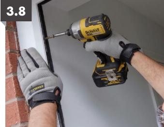
Install your first fixing on the latch side, fixing can be made either above or below the latch. Remembering to drill a 5mm pilot hole in the frame before fixing to the brickwork
