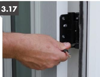
If hinge adjustment is required, the hinge can be moved left to right using the side hinge. Quarter of a turn should be sufficient, ensure that the top and bottom are both adjusted inline with each other on each hinge
