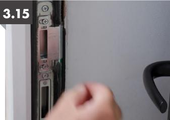
Check the tension on the door, pull the door closed so it latches and ensure there is no movement on the door. If you need to adjust the centre latch, undo the two screws which will allow for the centre catch to be moved in or out. Once adjustments have been made, repeat the process of closing and latching the door until there is no movement on the centre fixing.
