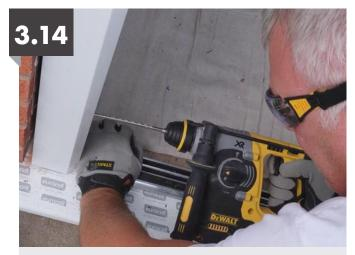
Install the remaining fixings, on both the hinge and keep side of the door, there should be 6 fixings in total on either side, with a fixing above and below each hinge and keep. Ensure a 5mm pilot hole is drilled in the frame prior to fixing to the brickwork.
