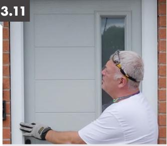
Bring the door slab to the fame checking that it touches top and bottom before the centre fixing is installed
