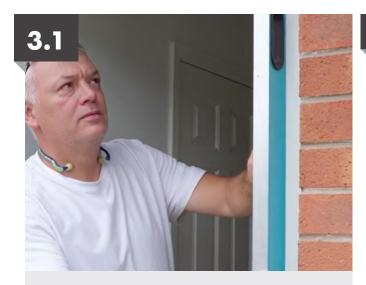
Install the hinge side of the frame plumb and level using a 6ft level/straight edge ensuring that the frame is packed (if required) to allow the head to be fitted level. Ensuring the hinges are centre, make sure you have a 4-5mm equal air gap between door leaf and frame from top to bottom.
