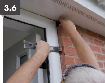
Using a crowbar to move the frame over, insert a 4mm/5mm packer at the top of the frame. This is to stop the frame from pulling over when the next phase of fixings are installed. This ensures an equal air gap between the two brush piles.
