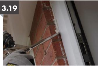
Expanding foam should now be applied between the frame and brickwork ensuring only enough is used to avoid distorting the frame when it expands. Once the foam has dried it can be cut away and perimeter sealing can be carried out. Ensure the frame is free from dust and debris before applying silicone. Do not seal across the front of the aluminium threshold as the drain holes are concealed behind the front ramp.
