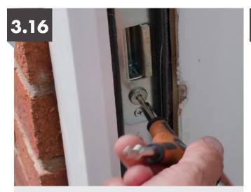
With the door closed, check the top and bottom of the door to ensure there is no movement. If you need to adjust the top and bottom latches, they can be adjusted using a 4mm allen key
