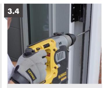
Install next fixings below the middle and bottom hinges, ensuring that a 5mm pilot hole has been drilled before fixing to brickwork.
