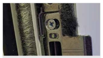
The top and bottom keeps can now be adjusted in the same way but the hooks should hit the plates so that they just pull the sash into the gasket slightly.
