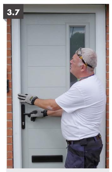
Pull the door slab up to the brush pile ensuring that it touches top and bottom
