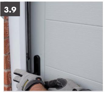
Bring the door slab to the fame checking that it touches top and bottom before the bottom fixing is installed
