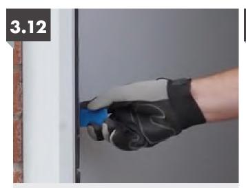
For the centre fixing on the latch side, place a 2mm packer between the frame and the plaster line, this will cause the frame to slightly bow outwards, which allows the centre catch to click in and the mechanism smoother to operate. Install the centre fixing remembering the 5mm pilot hole
