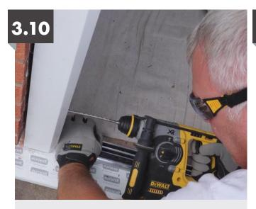
Install the bottom fixing, again remembering to drill a 5mm pilot hole in the frame before fixing to the brickwork
