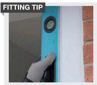
Remove the rubber from your level and get it right into the top when squaring up, you may find the frame is bending inwards in the top corner. This bending in of the frame causes issues with the way the sash hangs square.
