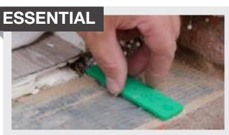
Always put a **4mm packer** under the hinge side leg. If the lock side needs lifting or dropping to square up the head you now have some room for that adjustment. Also seal with silicone between the threshold and cill to stop water ingress.
