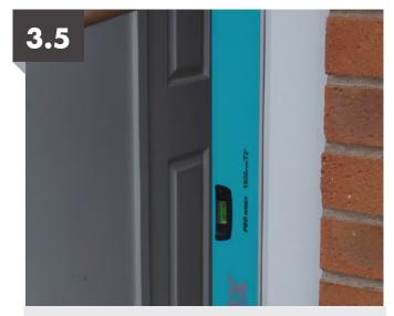
Place the 1800mm level on the frame and ensure that the frame and the level meet the entire way down the frame
