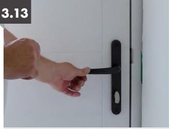
Now the centre fixing is in place, close the door to check the door closes and latches correctly.
