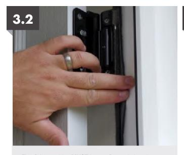
First fixing position **MUST** be two fingers below the top hinge. **Drill a 5mm pilot hole for each fixing before fixing to brickwork to avoid cracking the frame.**
