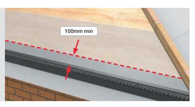
Starting at the right hand roof edge roll out and fix to the plywood roof panels EnvirolayFR® (ENVIROLAY) to the full roof face, fixing and securing the roof underlay at 450-600mm centres with clout nails as you go along. Overlap the universal eaves/ support tray by a minimum distance of 100mm.
