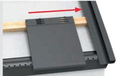
Take a new tile and clip into the starter rail, hook over the batten, then slide this tile into the end tile so that the connecting strip fits into the left hand slot of the tile. Push together ensuring there is a 5mm space between the top faces of the tiles.
