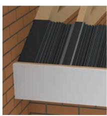
For abutment walls install the rafter roll out tray and fix to the end rafter
