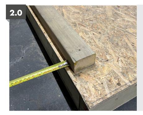
Install the side wall base plates 11mm in from the edge and centrally on the floor (to leave room for front and back panels) ensuring they are parallel to the side of the base.
