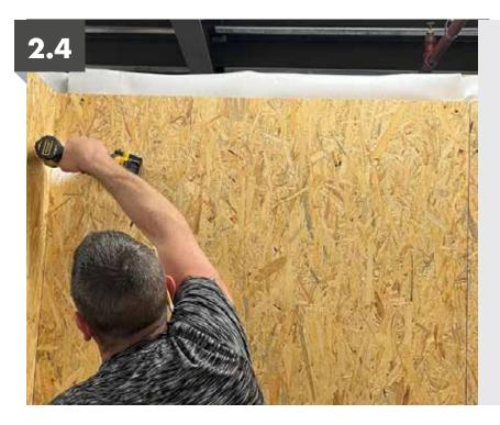
Where the panels meet screw from the inside to secure them together both vertically and along the base plate.
