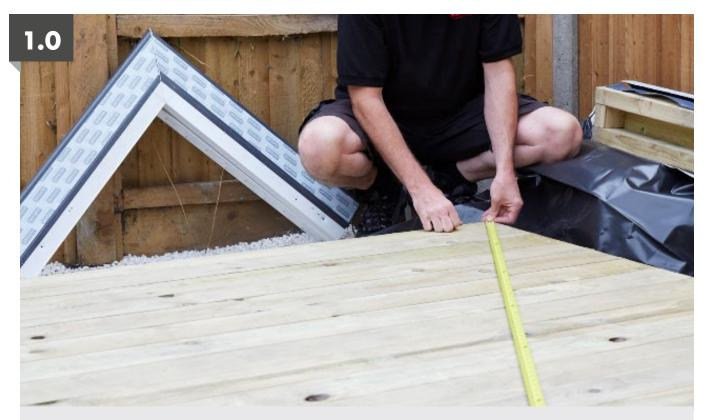
Ensure the base is clean and level. Take care to sweep away any loose gravel etc as this can prevent the floor panels slotting together.
