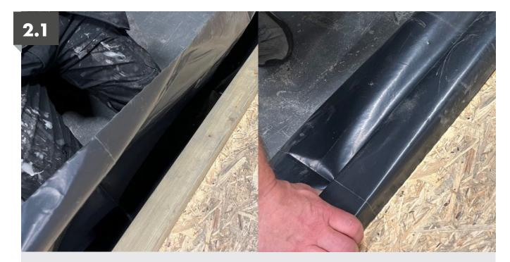
Fold the Damp Proof Membrane over onto the floor (this can be trimmed back later).
