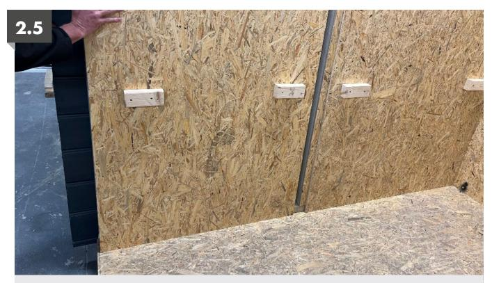
Continue to fit the remainder of the wall panels. The side and back panels slide together as shown below and are also secured either side where they join both vertically and along the base where they meet the base plate.
