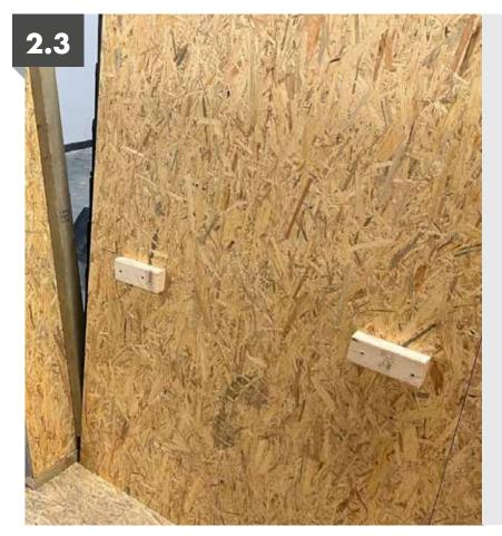
Lift the rear corner panel into place and slot it into the side panel.
