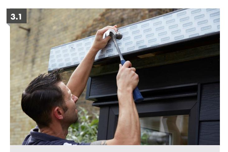
Fit the larger fascia boards to the roof as shown above using the poly pins provided. The top of the fascia board should align with the top of the roof at this stage.
