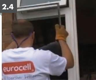
Remove as much glazing as possible, this will help to reduce the weight and allow easier handling.
