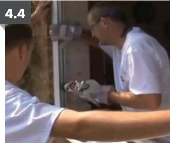
Check that frame is both level and plumb, then drill fixing holes into the frame sides. These should be drilled approximately 150mm from the top and bottom corners and approximately 600mm in between (a minimum of 2 fixings per side).
