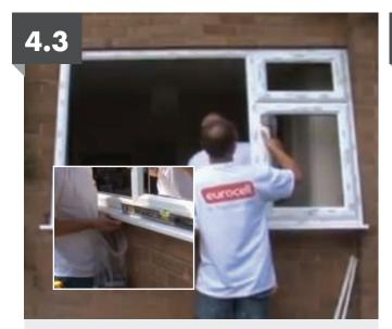
Carefully position the new frame into the aperture. Centralise it and insert packers underneath to level it and maintain the 5mm expansion gap.
