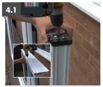
Remove any packaging from the new frame. Apply a bead of silicone along the length of the frame where it will meet the cill.
