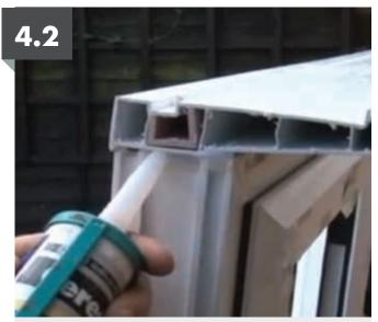
Be sure to seal the ends of cill and frame assembly to prevent moisture from tracking along the cill and into the brickwork.
