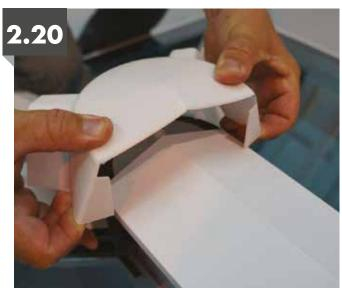
Splay the top cap and lower onto the ridge whilst checking the capping is positioned correctly over the rafter and hip top caps. The capping returns should clip under the ridge profile when positioned correctly.
