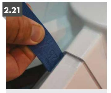
Ensure the capping is seated down correctly and remove any excess sealant from all edges.
