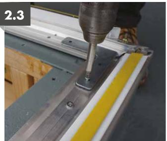
Fix the adjacent ring beam ensuring the joint is tight. Remove any excess sealant and secure corner using a steel corner cleat with 4-off 4.8x25 LG screws (supplied).
