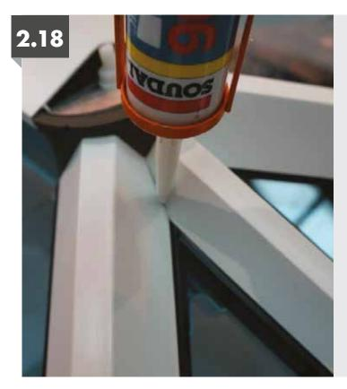
Seal the rafter top cap to hip top cap from the gasket intersection to foam bung.
