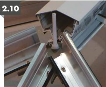
Locate the nylon bar through the spider and lock off using nuts and washers either side of the spider. The nylon bar should sit 5mm below the crest of the ridge profile.
