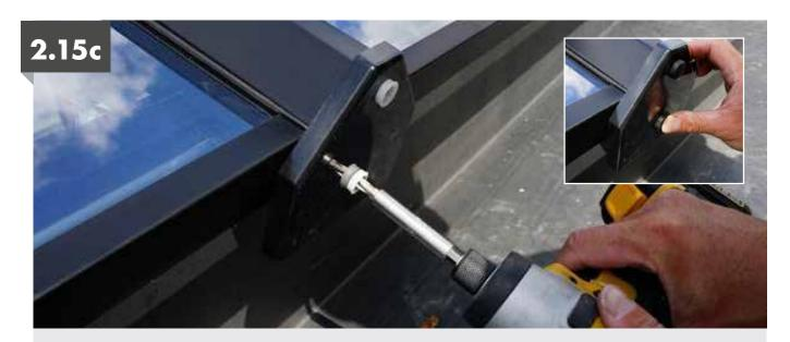
Protective film can now be peeled off and then glazing stops plus end plus end caps fully tightened and secure.
