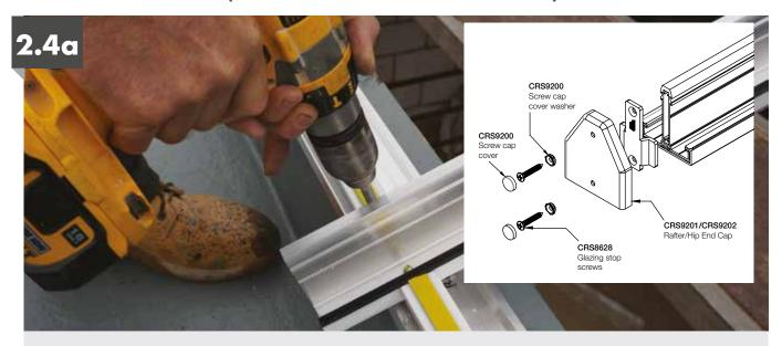
It is advisable to partially fit the glazing stops and end caps as shown (right) before fixing rafters to the ring beam. **Install the glazing** stop screws to approx. half their length, do not install screw cap covers at this point. You can then proceed to loosely secure the side rafters to the ring beam using the threaded studs located down the ring beam.
