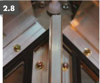
Fasten the central rafters to the spider using 1 x CRS8625S double stud and nuts. If jack rafters are present, please refer to Section 3: Installing Jack Rafters on page 13.
