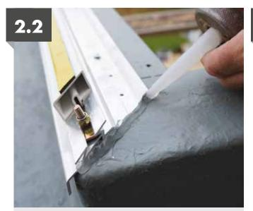
Run a bead of silicone sealant along the mitred edge of the ring beam to seal the corner joint, when the next ring beam is offered up.
