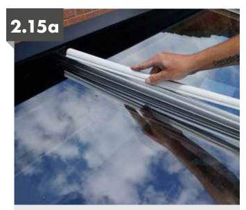
Ensure thermal breaks are installed on all glazing bars before attempting to install aluminium top caps. Do Not attempt to install the top caps with the thermal breaks with in the top cap as this will damage the top cap.
