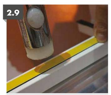
If not already fitted, clip in the eaves beam seals between the rafters and hips using a nylon mallet. Check the rafters are all square to the ring beam and ridge, and then tighten all roof fixing nuts.
