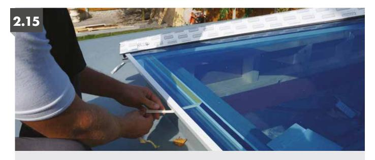
Fit the rafter and hip top caps using a nylon mallet, then ensuring the glass is positioned correctly, peel the remaining eaves beam seal tape film away and press glazing down to ensure contact with eaves tape.
