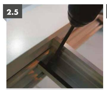
Supporting the ridge, the rafter bars can be secured to the ridge using the threaded studs. Once opposing rafters have been secured the ridge should be self supporting.
