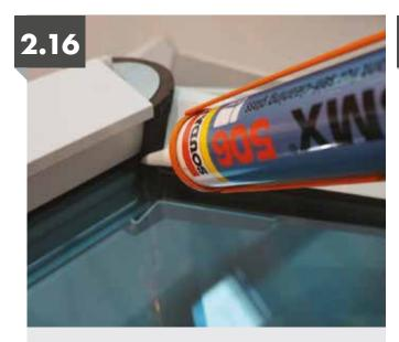
Seal around perimeter of the foam bung where it intersects the ridge glazing seal, glass and glazing bar top caps.
