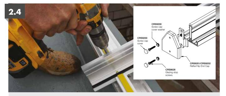
You can then proceed to loosely secure the side rafters to the ring beam using the threaded studs located down the ring beam.
