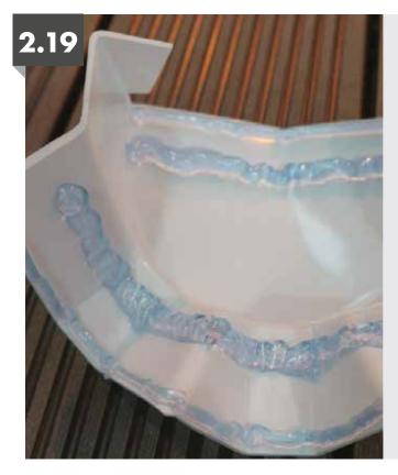
Using a suitable high-grab adhesive sealant, run a small bead on the perimeter edges of the top cap and a larger bead further inboard as shown.
