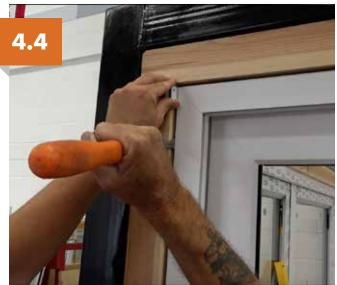
Pack the doors to keep it square and centralising the frame in the aperture and ensure it is level and square.
