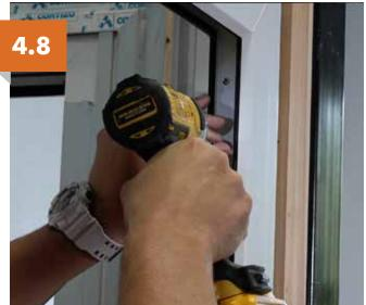
Remove screws from fixed sash and slide back away from frame.
