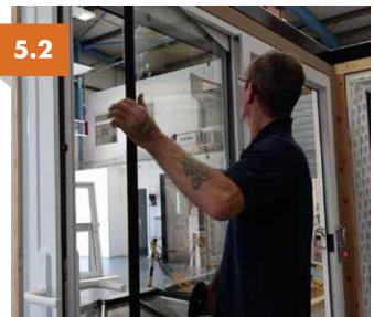
Lift the glass using a glass lifter, position lifter in centre of pane. Allow a slight angle on interlock side when offering up into position.
