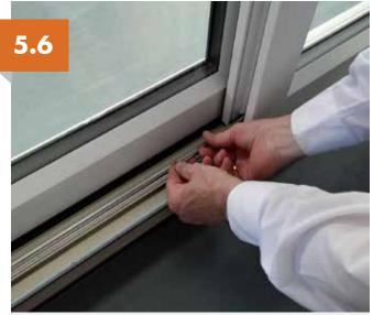
Adjustment – once the door is set, check to make sure the sash is square on the track. Use an allen key for adjustment of up and down movement if necessary.
