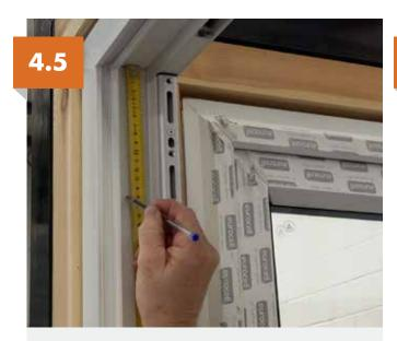
Open closing sash, mark 150mm from each corner of frame and at 600mm intermediate positions.
