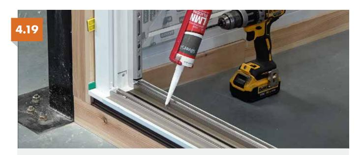
Mastic in the hole to seal the head of the screw.
