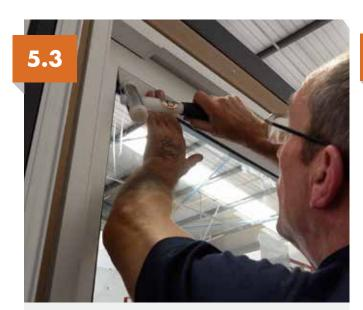
Pack glass to suit and put top/bottom beads into position first and then the sides.
