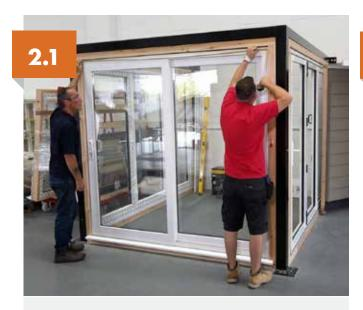
On arrival, before removing any existing door frames, check that the replacement frames size is the same as the existing door frames. When checking the sizes, ensure that the new frame has a 5mm expansion gap around the perimeter.
