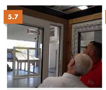
Check the operation for a perfect gap at the top and bottom of the frame.
