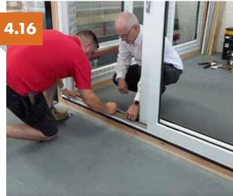
Mark position (again 150mm from the bottom corner, and the in 400mm increments) the bottom fixings into the base.
