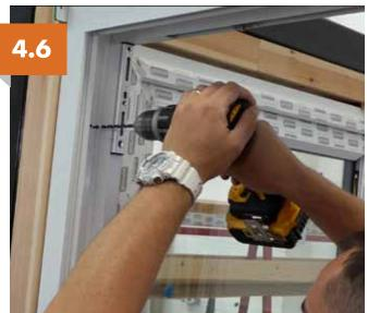
Drill clearance hole for relevant fixing.
