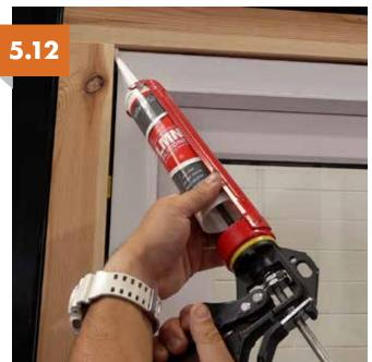
Silicone sealant using a low modular sealant to finish around the frame.
