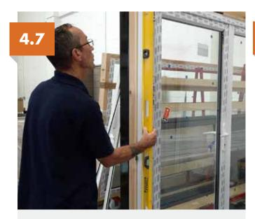
Check frame is plumb and level before any fixing.
