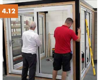
Slide sash back across and fix sash to frame.
