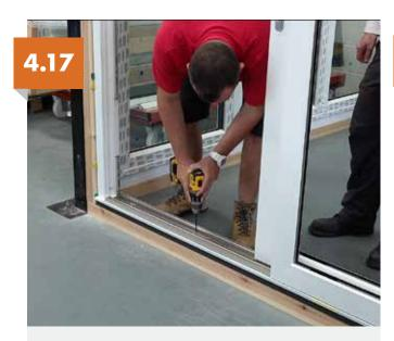
If the base is aluminium low threshold, be careful not to damage the thermal break. To ensure this doesn't happen, drill just behind the thermal break.
