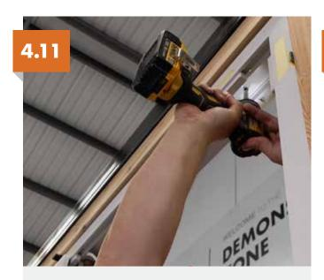
Peel trim down to fix underneath and then clip back into position.
