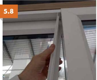
When 100% happy that the door is set, position the interlock covers in place. Tap the back in first down the length then tap down the front face.
