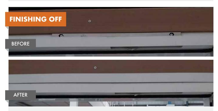
If desired, the soft close actuator can be covered, so that it is no longer visible. To do this you can fit a cloaking fillet C30 trim or similar to the head of the frame, from width to cover.
